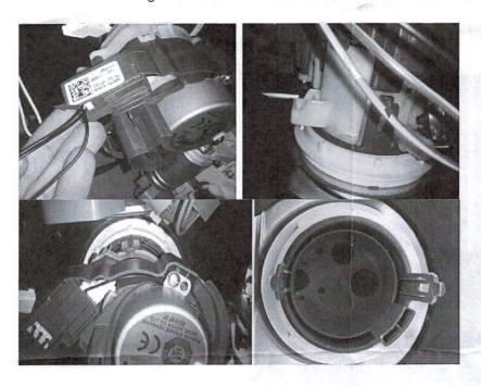
2. Install the insert. Insert is possible to install only in one position. Install it in sequence like on photo bellow (a click must be heard).
